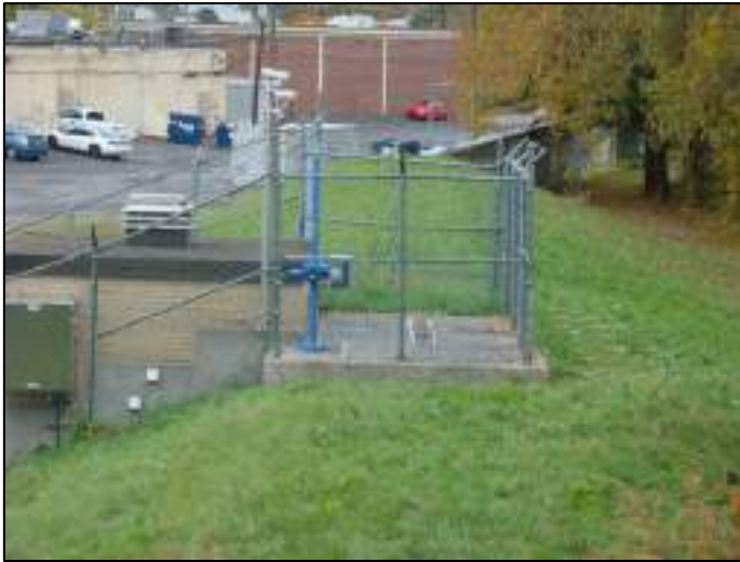
Figure 25: Army Corps of Engineers Levee behind Kingston Plaza from Col. Chandler Drive. This is the control gate to release water back to the Esopus if it collects behind the levee. - Photo by Gregg Swanzey
