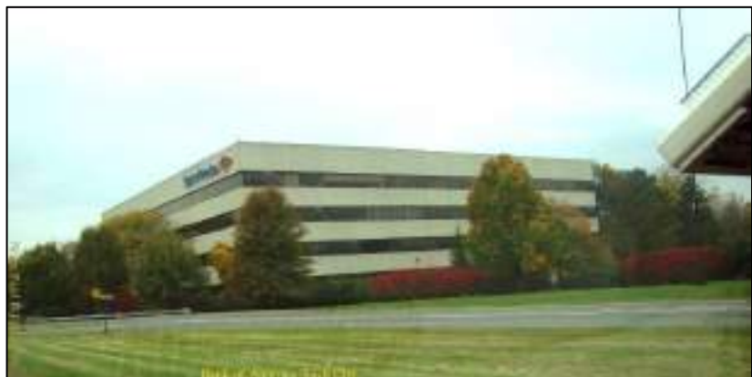
Figure 33: Bank of America in Tech City - Photo by Nora Budzjak
